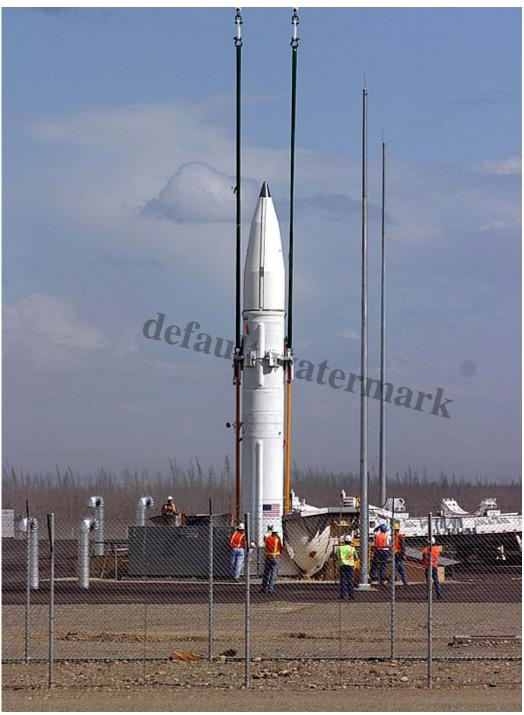
A <u>Ground-Based Interceptor</u>, designed to destroy incoming <u>ICBMs</u>, is lowered into its <u>silo</u> at the missile defense complex at Fort Greely, July 22, 2004.
