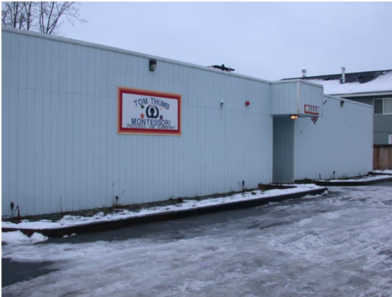
TTMS East on Boniface near 24 th Street
