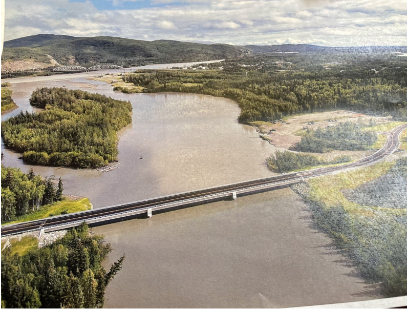
The New Nenana Bridge to Totchaket
